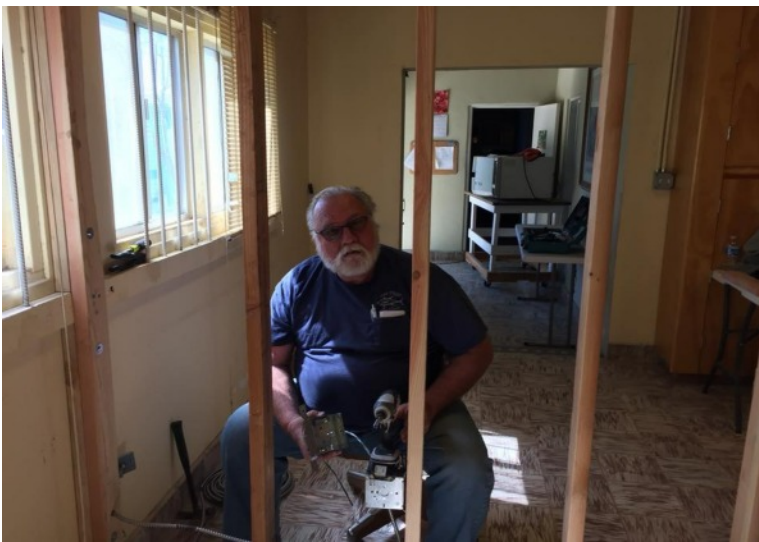
Richard Lenyk has worked for months on the renovation of the old and new optical clinic
